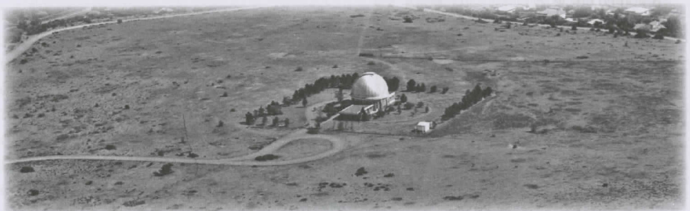
Figure 2. Aerial view of Lamont-Hussey Observatory and surrounding game reserve, 1954. (Lowell Observatory Archives)
